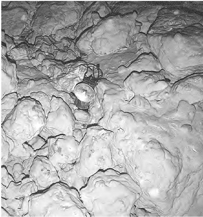
Photo 12: A rubble mound in the intertidal zone of CI-10 that is cemented and coated by calcite deposits.
