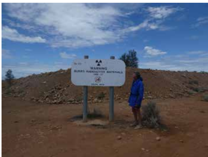
Figure 8. Debris capping over shallowly buried contaminated materials at the Taranaki site.
