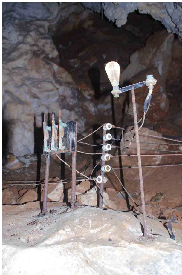
Figure 1. Electric lighting from the 1880s still in situ, Off the Track tour, Jenolan.
