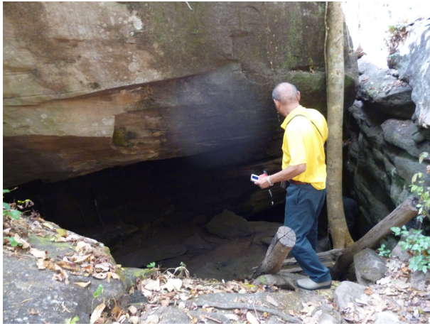
Fig. 33. Tham Seri Thai rock fall leading to stream.
