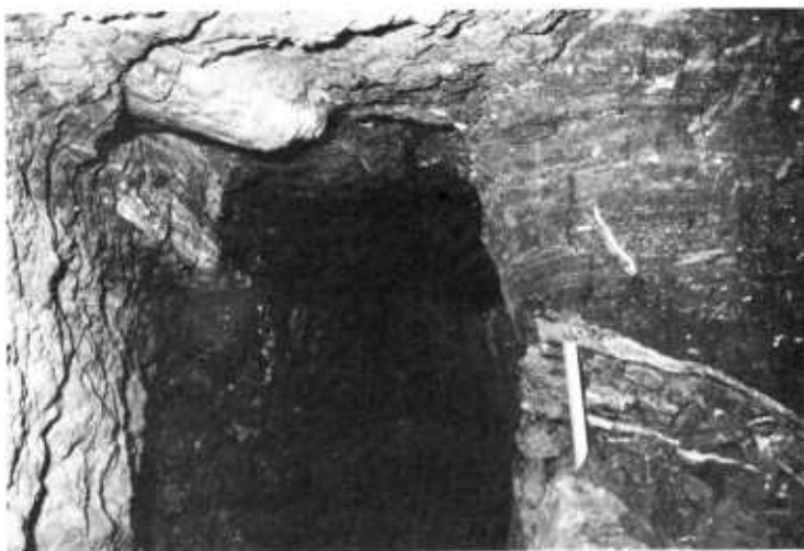
Plate 3 Units 1 (BG), 2 (FS) and 3 (RB), Phosphate Mine, Wellington. Scale is 30 cm long.
