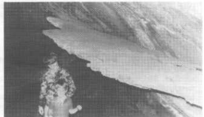
Plate 8: The Table - a thin sheet of lining near the entrance to Pinwill Cave showing a degree of plastic deformation. Photo: V.G. Atkinson.
